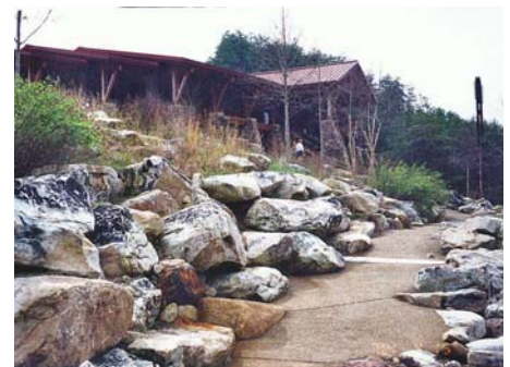
Ramp hardened with boulders
