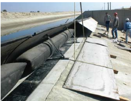
Obermeyer gate with shield cover
