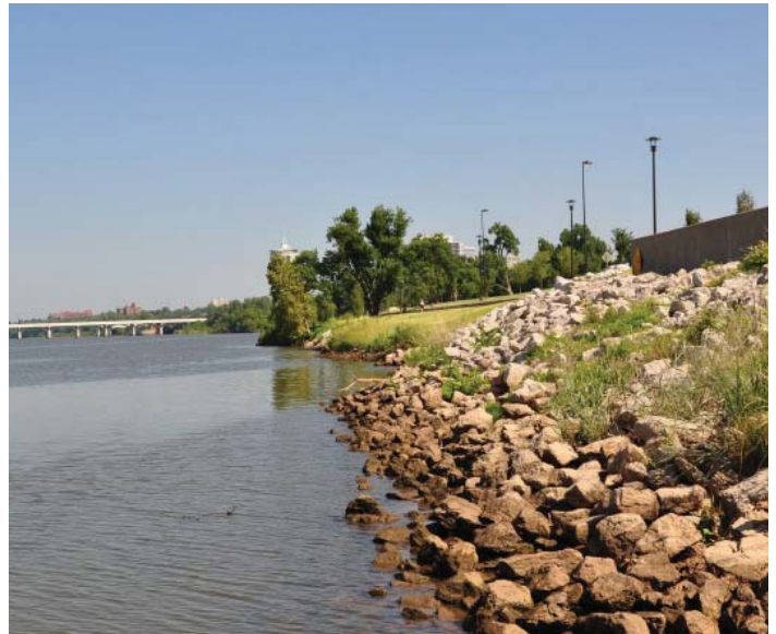
Bank stabilization upstream of the Zink Dam (east bank)
