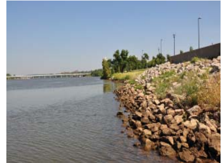
Rip rap stabilization near Zink Dam
