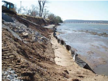
Rip rap bank stabilization near 41st St.
