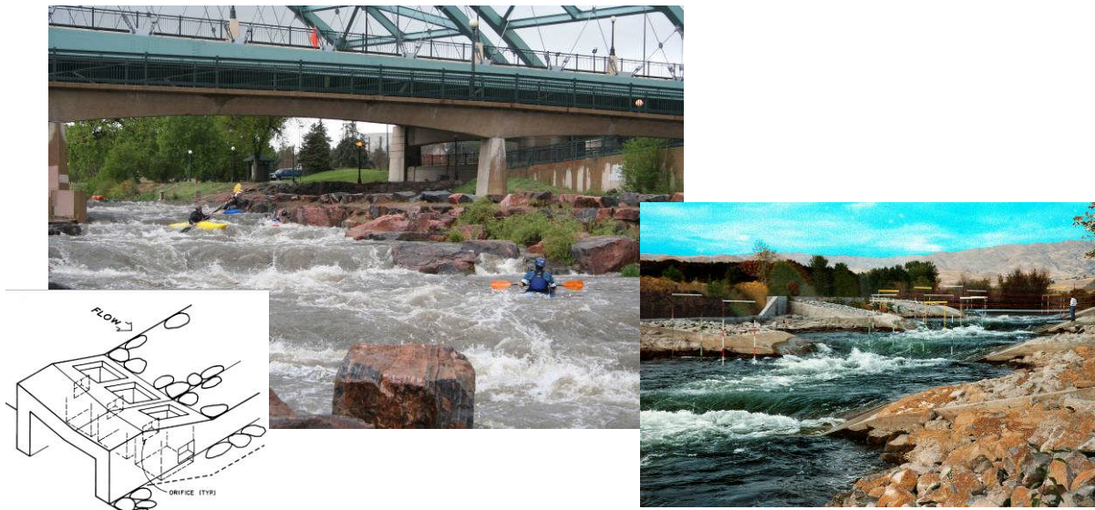
Roughened Channel Fish Passage is Integrated in these Multi-Purpose Recreational Projects.
