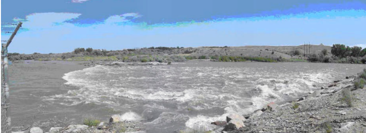
Sloped Face Spillway at the “Hogback” in New Mexico (Bureau of Reclamation) Designed for Safety and Fish Passage
